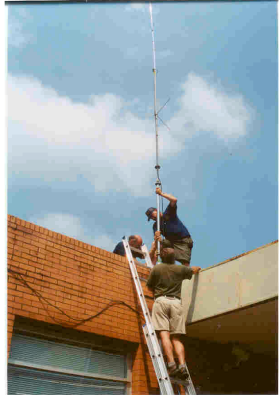
Vern, James, & Kenny mount ARX2B and prepare to raise 30' push-up pole.
